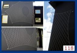
CABLETECH® Flexible Nets act as membrane. The net itself is formed in an area from the basic right-angled rectangular mesh without cutting and clipping together. It is due to fact that the shape and proportions of the individual mesh continously varies depending on the distribution of forces within the membrane.
